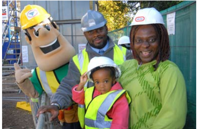
Ivor Goodsite shows local Neasden family around the building site at Ebony Court
